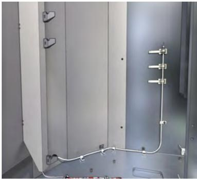
3. Carefully extract the temperature probe through the slitted bung.
