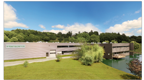
interscience R&D center and manufacturing plant Mourjou FRANCE
